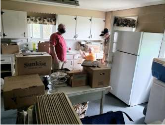
Emptying the kitchen so renovations can begin.
