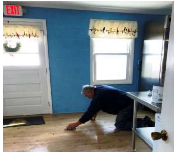
Constant clean-up needed during renovations.
