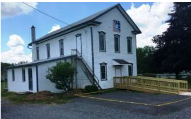
Accessible entrance ramp & handicap parking
