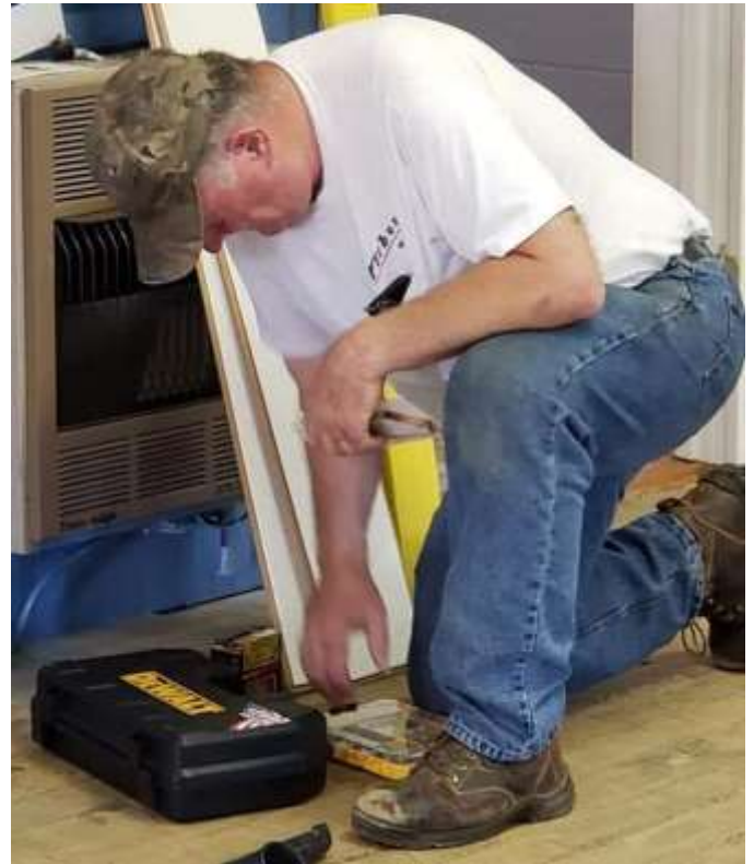
State Grange President Wayne Campbell joined volunteers to help with renovations.
