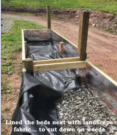
Next layer is gravel... for drainage
